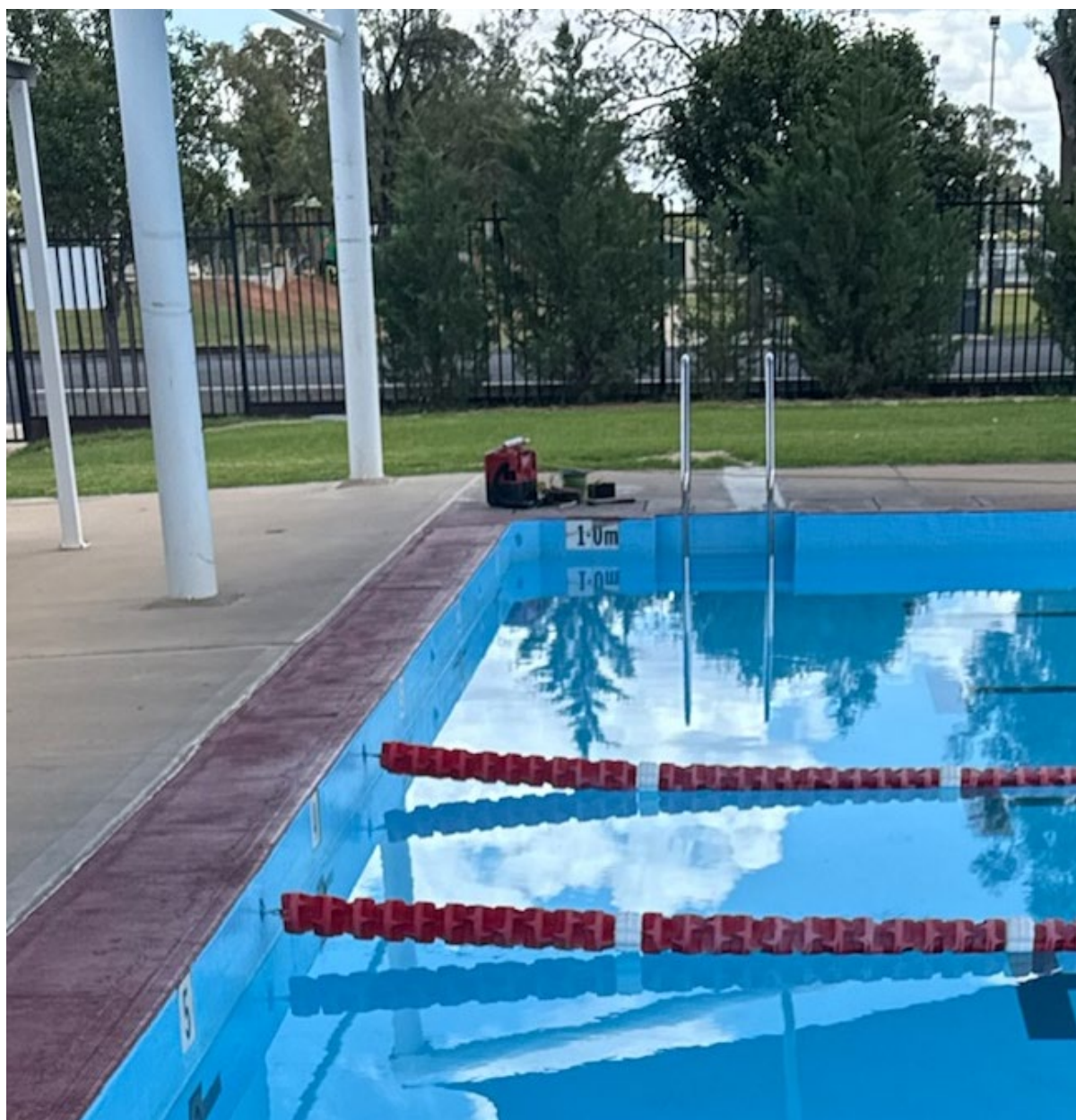
Figure 1: New handrails have been installed at the Trangie Pool
