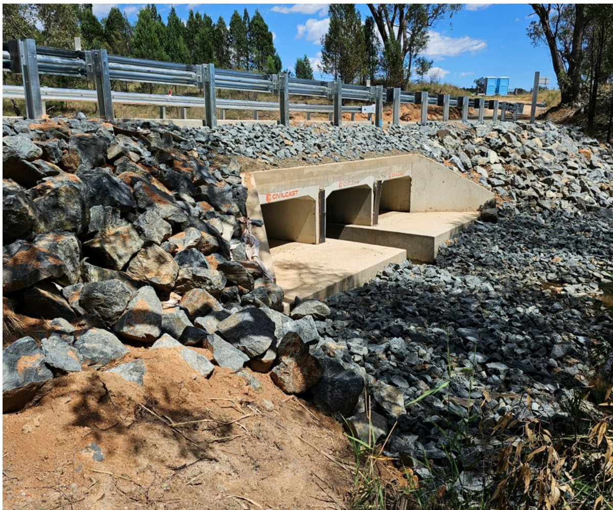
Figure 5: The culvert structure on Momo Road is now complete
