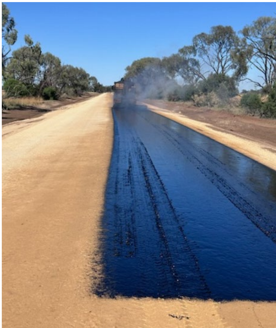
Figure 4: Sealing works on Enmore Road
