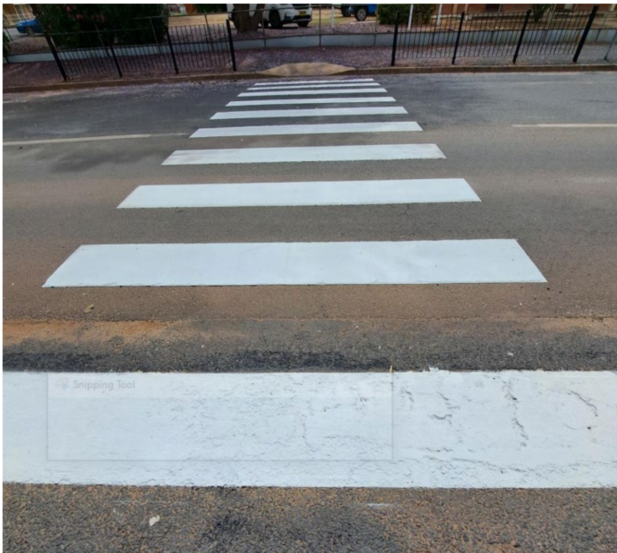
Figure 2: Transport for NSW completed works on the Dandaloo Street Pedestrian Crossing
