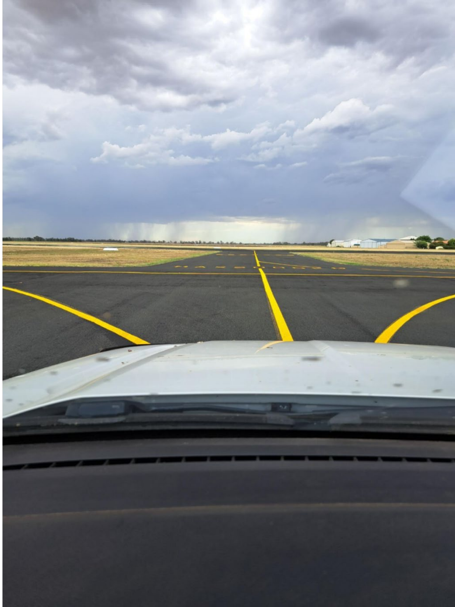
Figure 3: New line-marking at Narromine Aerodrome
